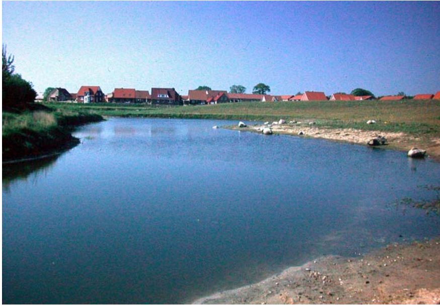
Fig. 6 One of the ponds shown in Fig. 5 right after excavating und flooding. On the accessible right side the shoreline was designed flat, on the left side steep to enhance biotope diversity.
